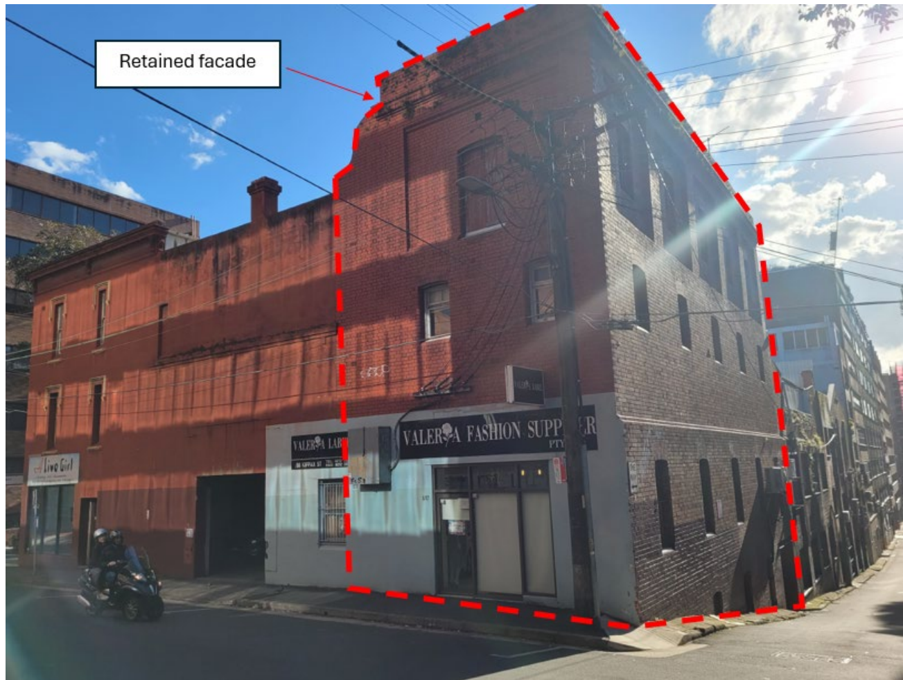
Site viewed from corner of Waterloo Street and Sophia Street looking south-west
