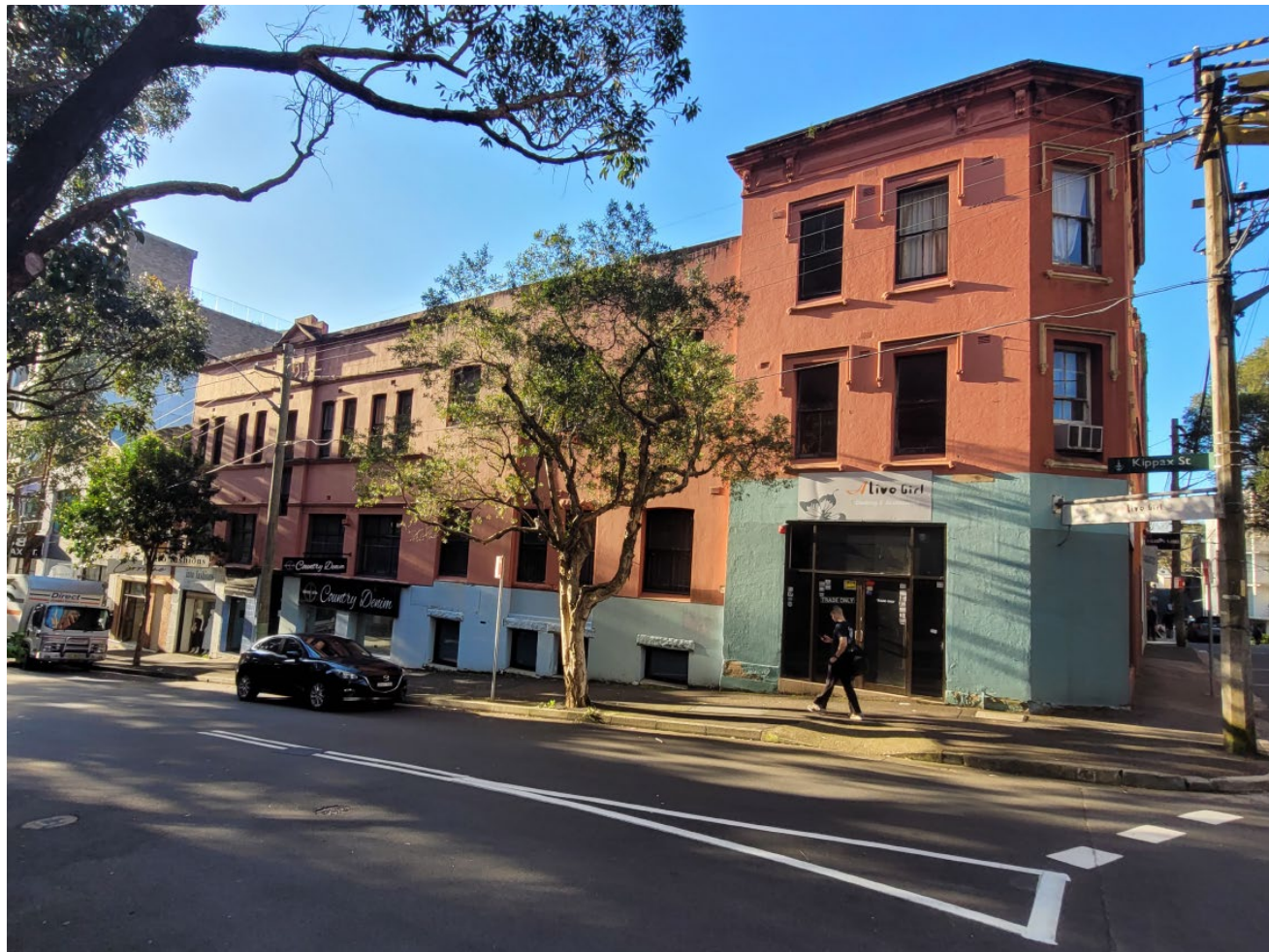
Site viewed from Kippax Street looking north
