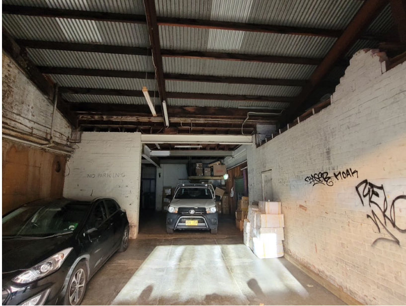
Existing loading dock
